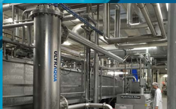
ARDO-FRIGODAN - DENMARK UV systems for recycled process water in the production of frozen vegetables
