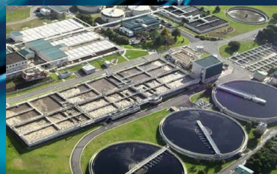
WASTEWATER, CROATIA Channel system for wastewater disinfection
